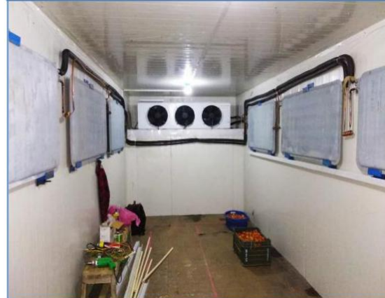
Fig 1: PCM based solar micro cold room installed at Mirge, Nepal
