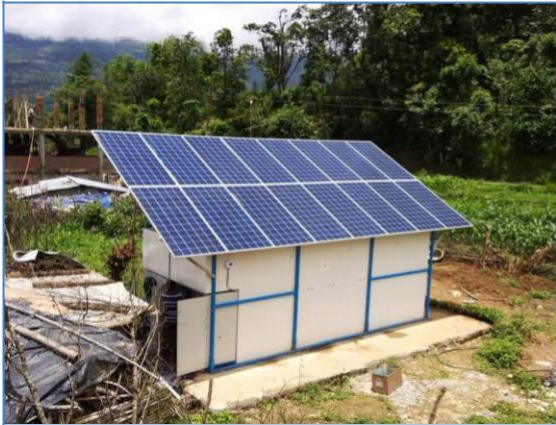
Fig 1: PCM based solar micro cold room installed at Mirge, Nepal
